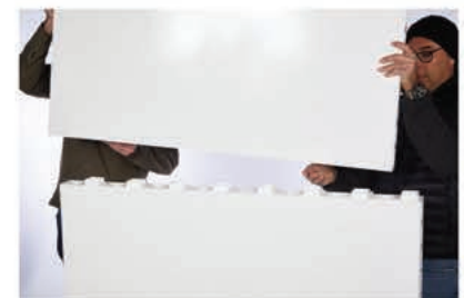
Placing a 2nd panel on top of a first EverPanel
