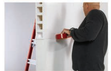
Placing construction seaming tape over seams before installing wallpaper
