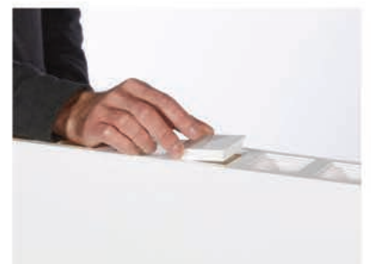
Installing Finishing Caps on an EverPanel
