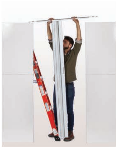
Positioning a Lintel with Accordion Door on top of EverPanels.
