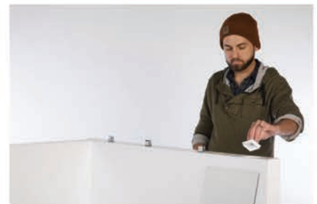
Installing EverPanel Mounting Caps
